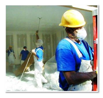
Drywall consists of a thin layer of gypsum between two layers of heavy paper. It is both faster and cheaper to install than plaster and is, therefore, widely used today in most buildings on both ceilings and walls.
